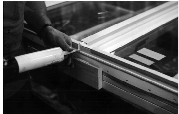
7. Apply silicone to the frame clad joints as shown in the photo.
